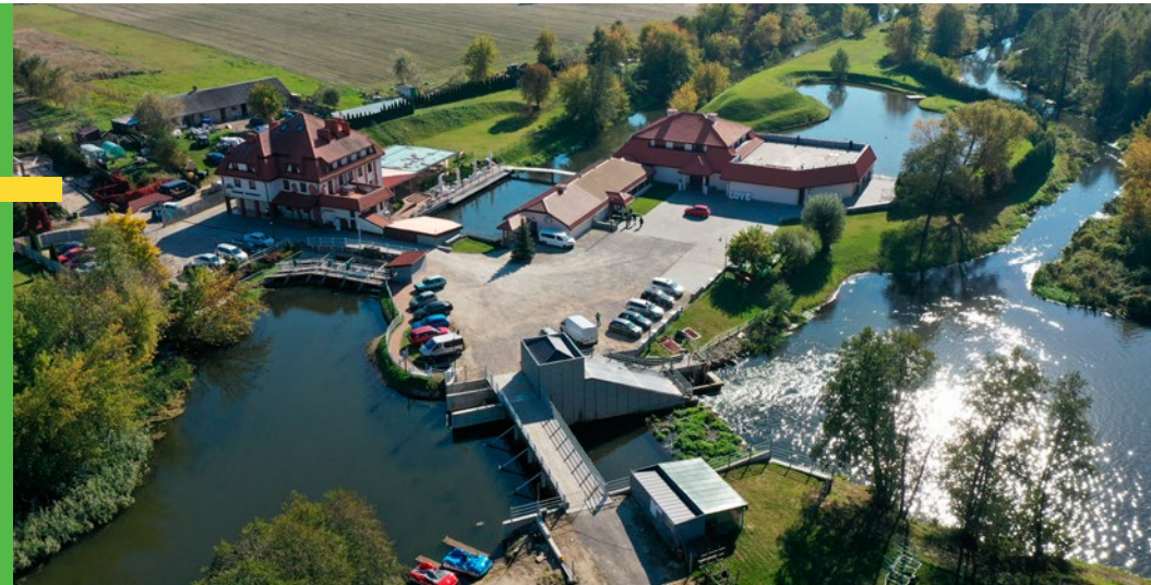
SHP Smrock, Poland – this is an example of ensuring the biological continuity of a river using an active fish pass, equipped with two Archimedean screws, the first operating in turbine mode and the second in pump mode.
